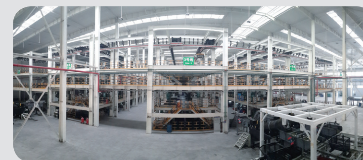
Threading, Air Pressure Test, and Anti-rust Treatment
